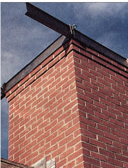
This steel crown form features integral clamps for fast and easy adjustment.
