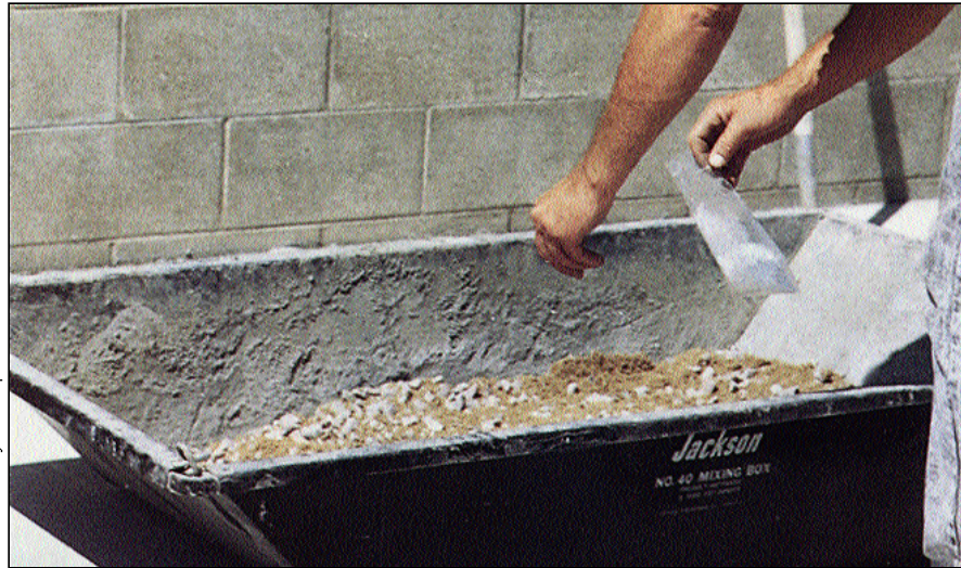
Integral fiber reinforcement may be added to the chimney crown concrete during mixing.
